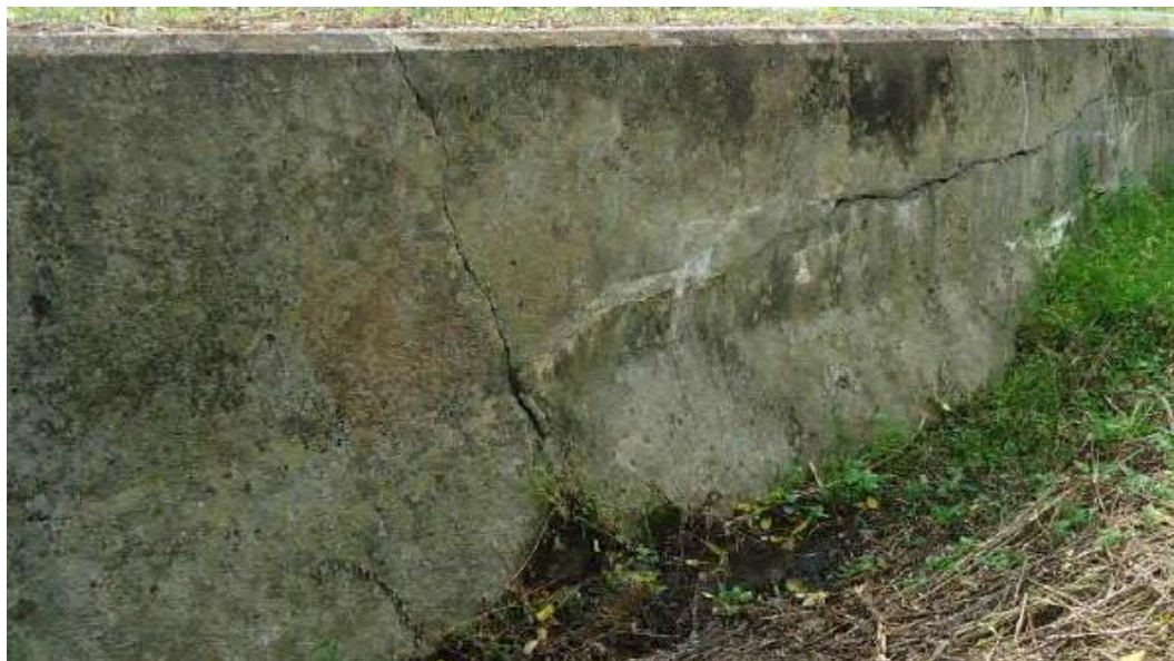
Figure 6 - Cracks 17
