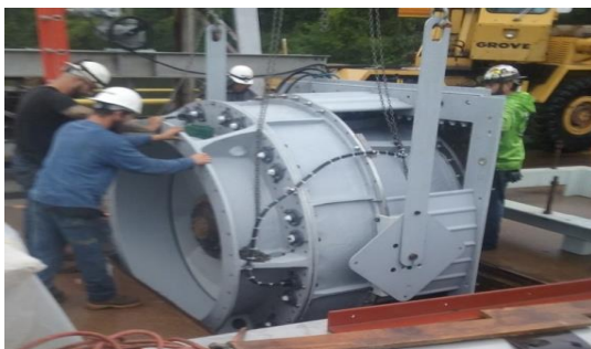
Figure 16 - ATS-63 all-composite turbine/generator installed in Mississippi dam, Brainerd, MN 38
